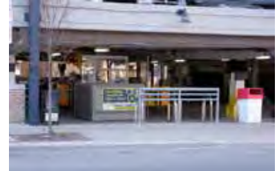
The bottom floor of the 4th & William Parking Structure along Fourth Ave.
